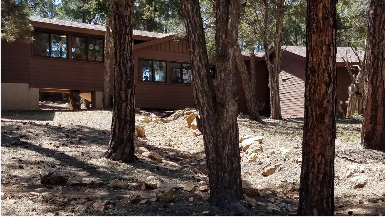
Figure 7: Example of channel on site (a)
