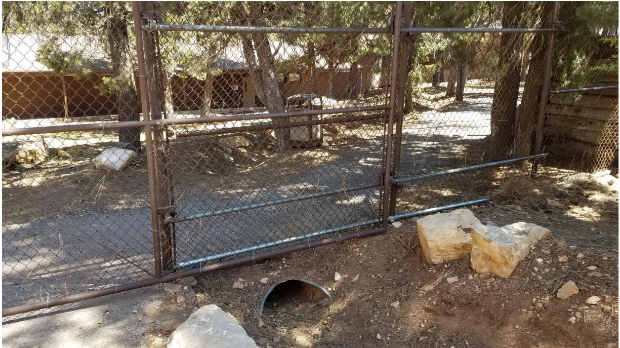
Figure 5: Example of Culvert on Site
